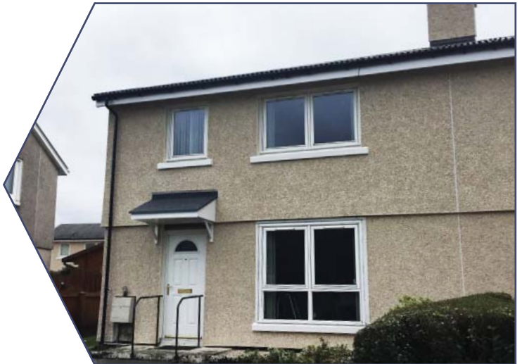
Over £1.8 million was spent on Major Repairs contracts in the year, including bathroom renewals, foyer refurbishments and external wall insulation (pictured)
