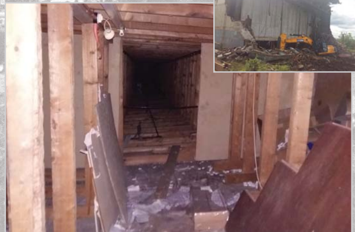
The original sloped cinema floor remained under the bingo floor
