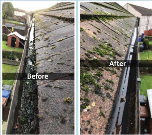
The gutters of these Kirkwood Avenue properties look great after cleaning
